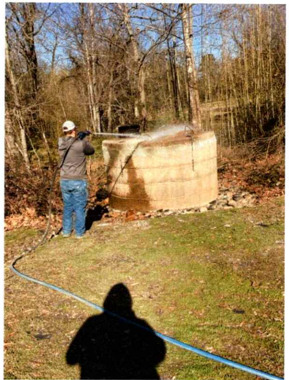
MH 1865 During cleanup
