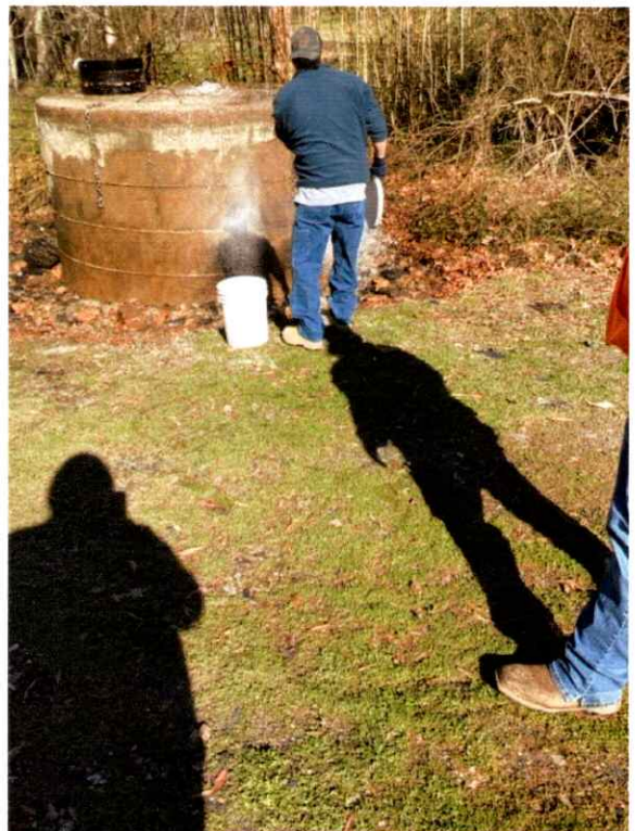
MH 1865 During cleanup
