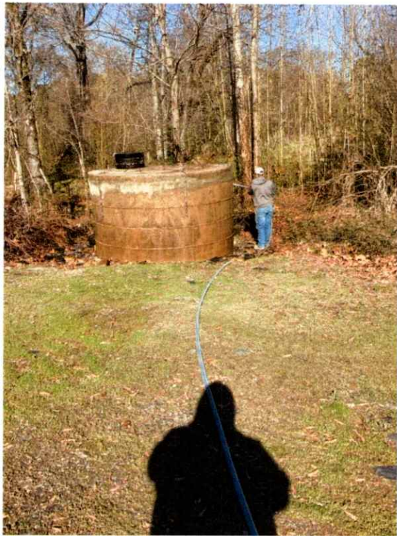
MH 1865 During cleanup
