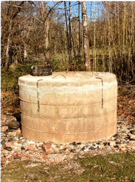
MH 1865 After cleanup
